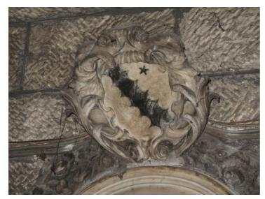
The crest leans forward but on site inspection indicates that it appears to be secure upon its original fixing.
